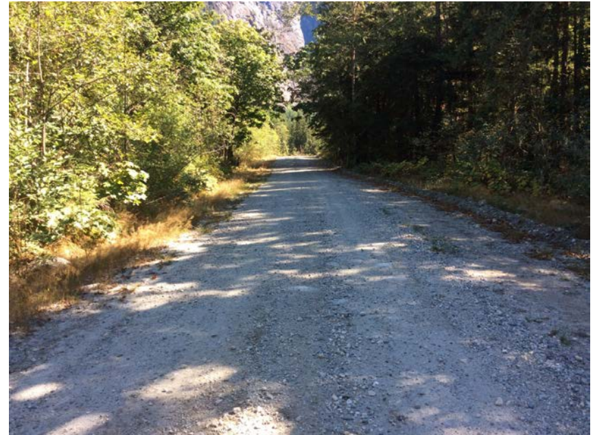
Left approach viewed from bridge
