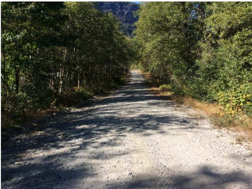
Right approach viewed from bridge
